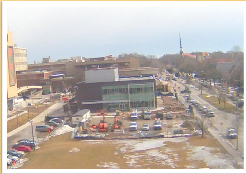
LECWC Construction Cam March 14, 2019
