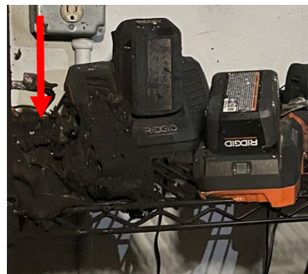
Picture: Rechargeable Battery Fire
