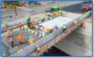
SR-1 Bridges, Delaware Waterproofing and strengthening UHPC overlay
