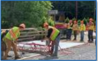
3 Bridges on RT 17B, New York Waterproofing and strengthening UHPC overlay
