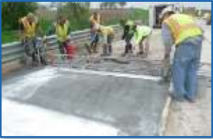
Mud Creek Bridge, Iowa First structural UHPC Overlay in the U.S.
