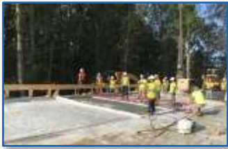
Blackbird Creek Bridge, Delaware Precast bridge-deck connections and waterproofing UHPC overlay
