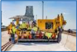
10 Bridges (DE, NJ, NY, IA, RI, IL) Machine laid UHPC overlays for bridge deck repairs
