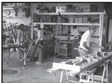
Friends of the Cedarburg Bog volunteers worked in the Field Station Maintenance Shop constructing boardwalk sections.
