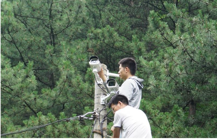
Fig. 3 On-the-spot installation of the Phenology camera
